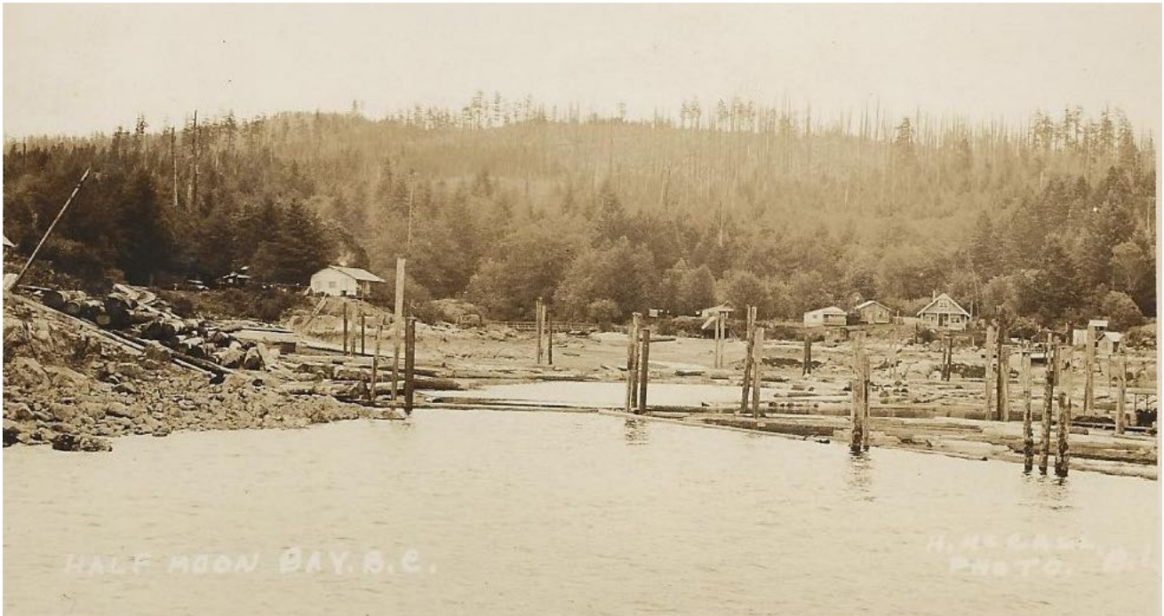
Halfmoon Bay in the early 1930s. The cottage on the left was supposedly the Tait's summer cottage. The gable roofed house with the white trim is the permanent home they constructed in 1931. Between the two the footbridge is faintly visible. Helen McCall photo. Source: Sunshine Coast Museum & Archives
