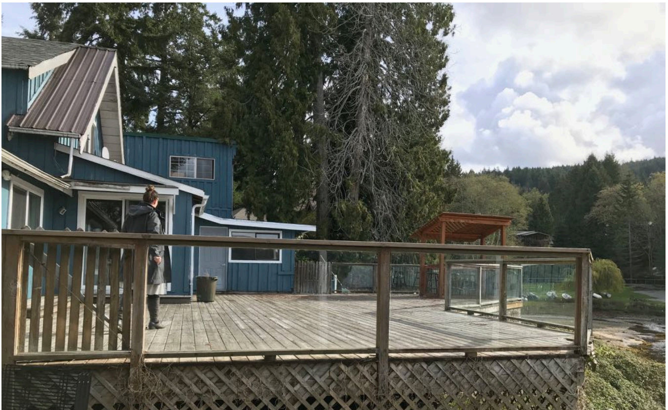
Below: view of the rear deck and rear of the store from the side
