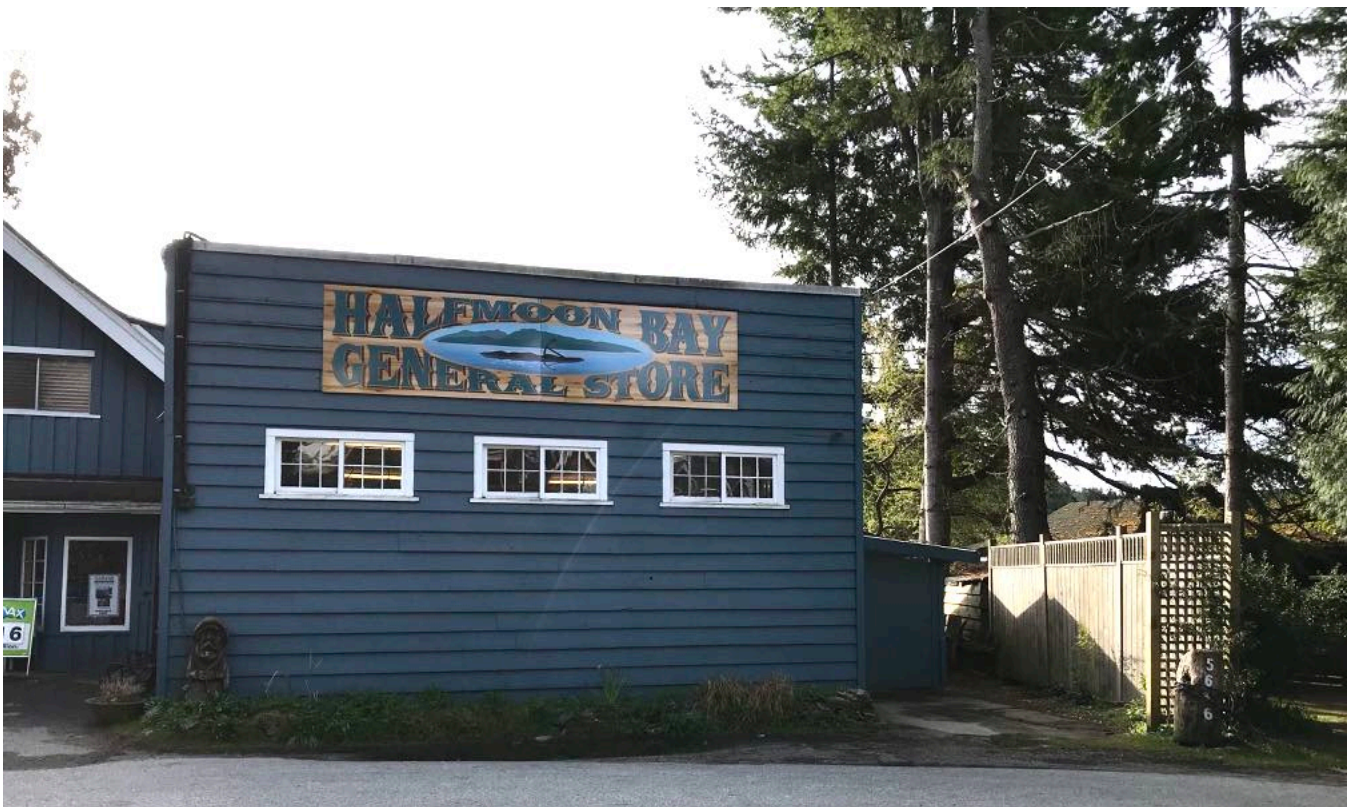
Below: front view of 1949 extension building, attached to the store building.
