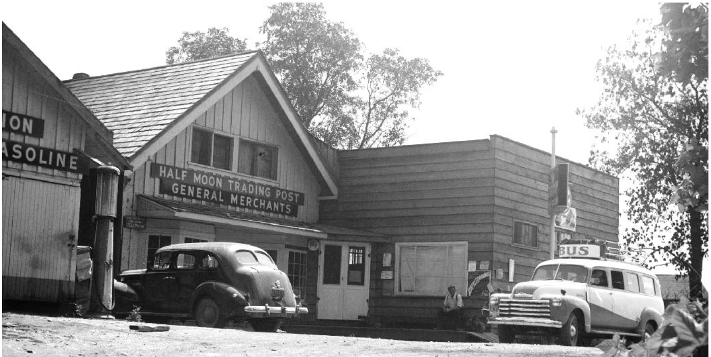
The store (middle), the warehouse/garage building (left) and the flat-roofed addition (right) built by Pratt in 1949. Source: Grant Hanney private collection
